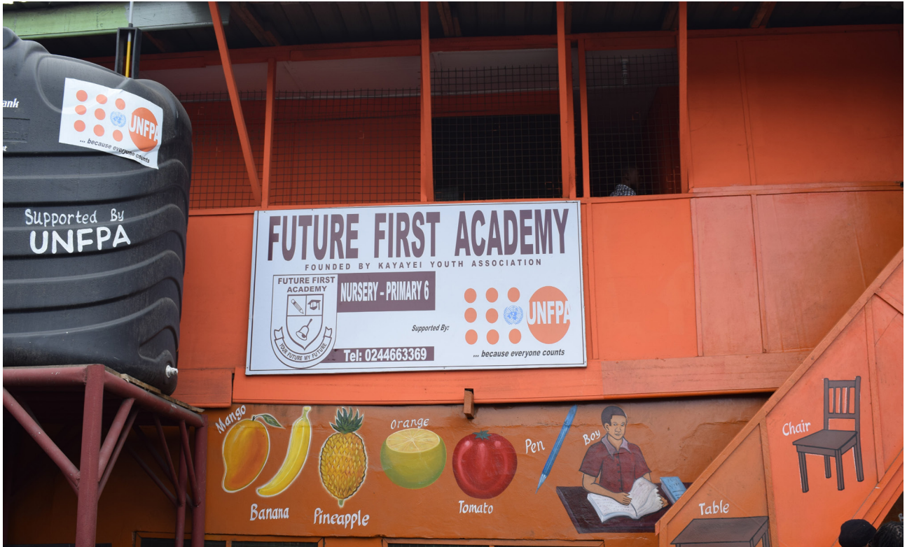
State of the Kayayei Children's School after refurbishment
