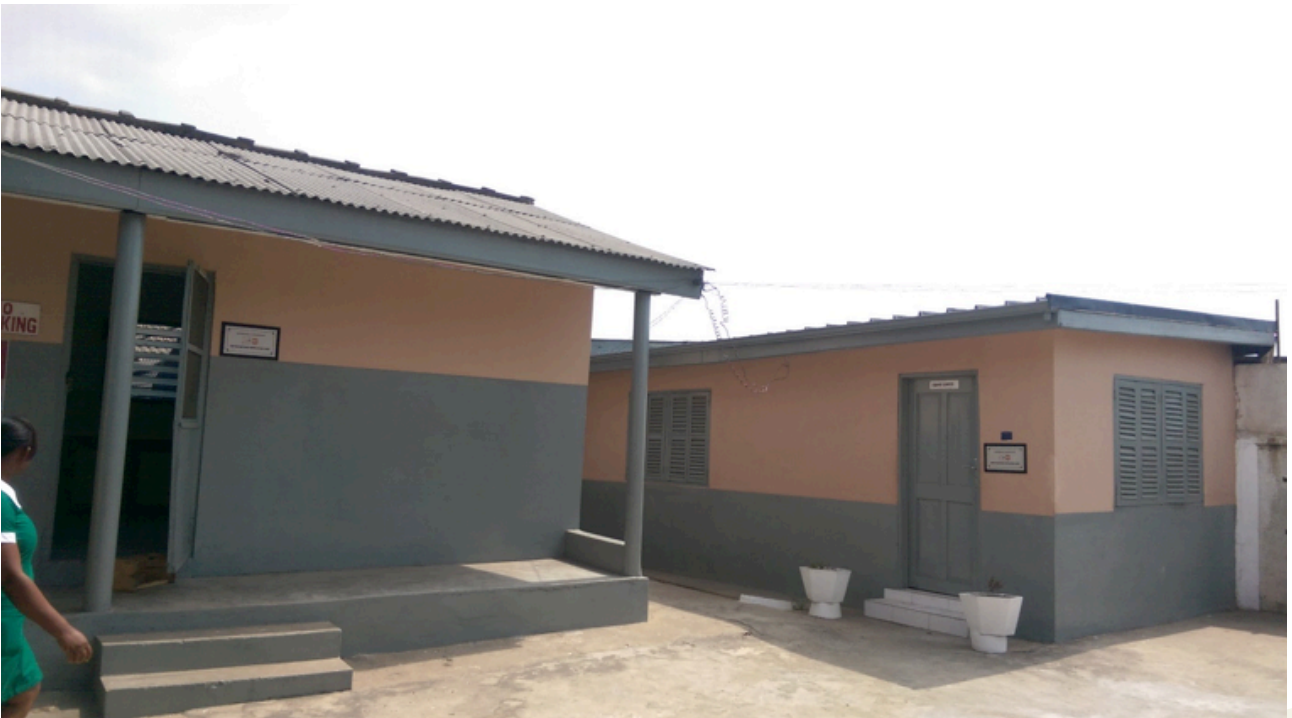
The Sewing and Nutrition Units after the renovation Photo credit: Claudia Donkor
